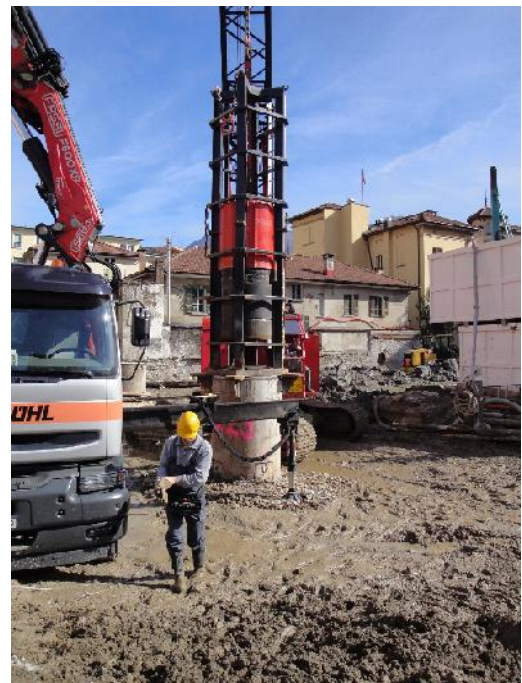
Figure 5. Dynamic Load Testing Equipment
